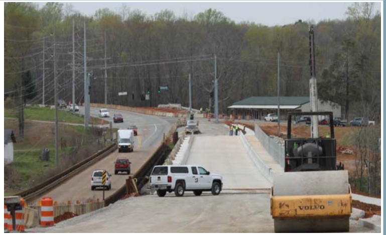
Winchester Road Bridge: old on the left, new on the right
