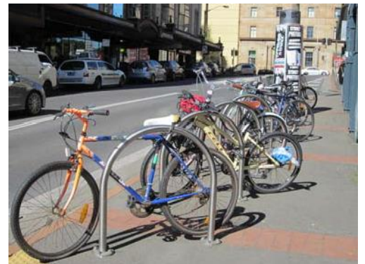
Figure 6: Metal rail secured to the ground designed for two bicycles per rail
