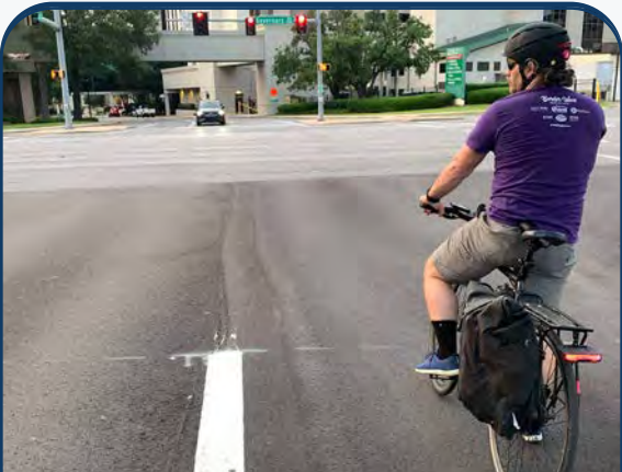
Recent repaving at the intersection of Governors Drive and Gallatin Street. As part of repaving efforts, check if bike detection symbols need to be repainted and the bike detection is working properly.
