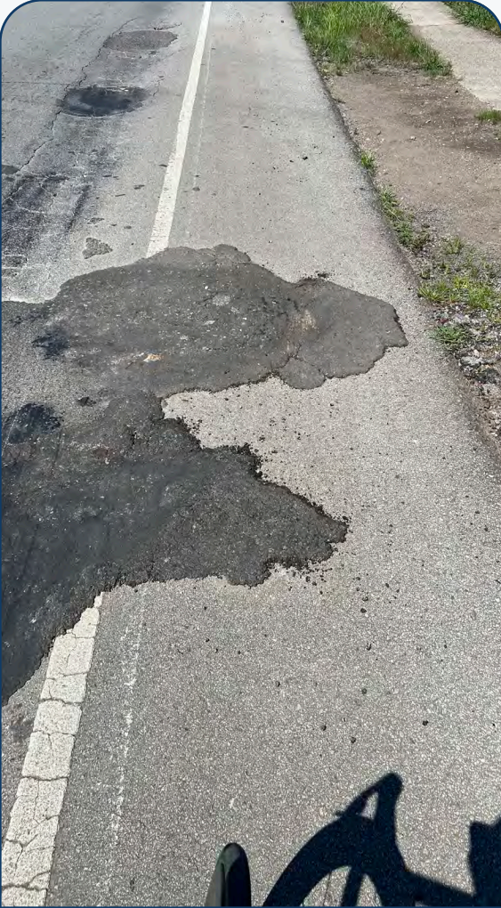
Uneven roadway patching can cause hazards for riders in the bike lane.
