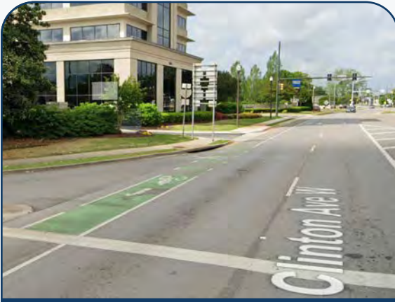
The green bike lane paint at the Clinton Ave at the Memorial Parkway Southbound ramp is worn and shows signs of repeated stopping and breaking. Bike lane striping will need maintenance on an as-needed basis, especially near intersections.
